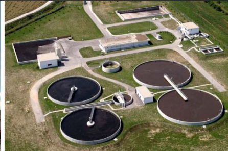
Waste water treatment plant construction
