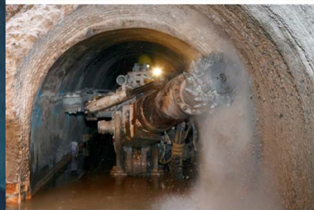
Trenchless pipeline rehabilitation
